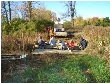
1. Repairing a bridge on a club trail
